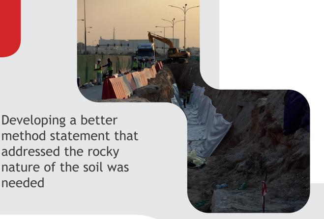
To help combat flooding, several projects were initiated in 2016/2017 across a bustling capital in the Middle east. The general scope of works included the design and construction of more efficient drainage network using larger perforated pipes, swale, and surface storage channels.
