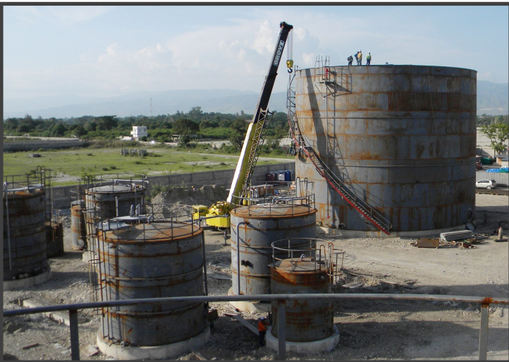
Construction of Tank Farm, Haiti
