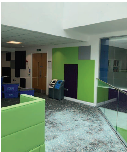
The above three images show an example of the incorrect glazing in the overhead position that has suffered Spontaneous Fractures due to Critical Inclusions. The images effectively demonstrate the safety implications of these fractures.
